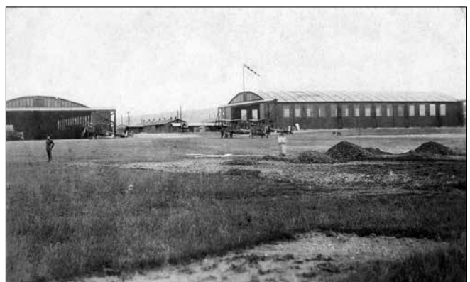
YATESBURY An RE8 and a pair of DH6s on the eastern No.2 aerodrome. The 1916 pattern GS sheds on that aerodrome were unusual employing a polygonal roof trusses with a flatter than normal apex.
