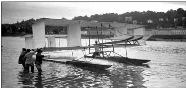
*Gabriel Voisin's glider fitted with floats made the first flight from water on 6 June 1905 towed behind a racing motor launch.* :Colin Huston
