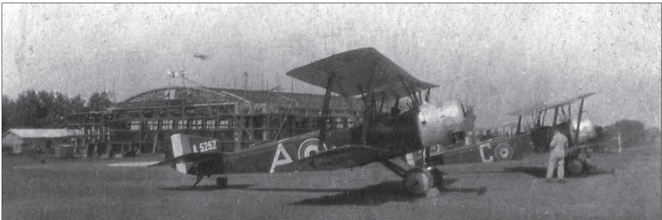
A pair of Sopwith 1 1/2 Strutters of the WEE at Biggin Hill, with Wells-built A5252 nearest. Both had the lower section of the engine cowling cut away and had their unit identity letters repeated on the fuselage turtle decking. The photograph dates from the summer of 1918, when the GS shed in the background was under construction on Biggin's south-west boundary (see GFS p.020 CCI 41/3).
