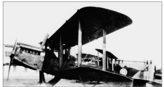
Airco DH4 B5510 had the 230hp Puma engine and was photographed on one of the permanent aerodromes on Salisbury Plain, probably its home base at Lake Down. Built by Vulcan, it came from the batch B5451-B5550 which was delivered during February and March 1918, too late for it to have been a 2 TDS machine. In addition to its station marking, it had a coloured fin, probably white and blue. :via M Davis
